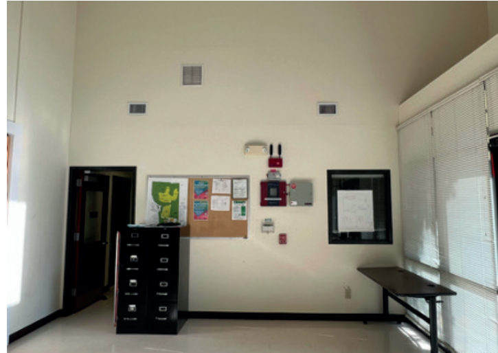
Lobby (facing classrooms)
