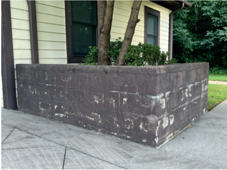
Front, brick wall, right
