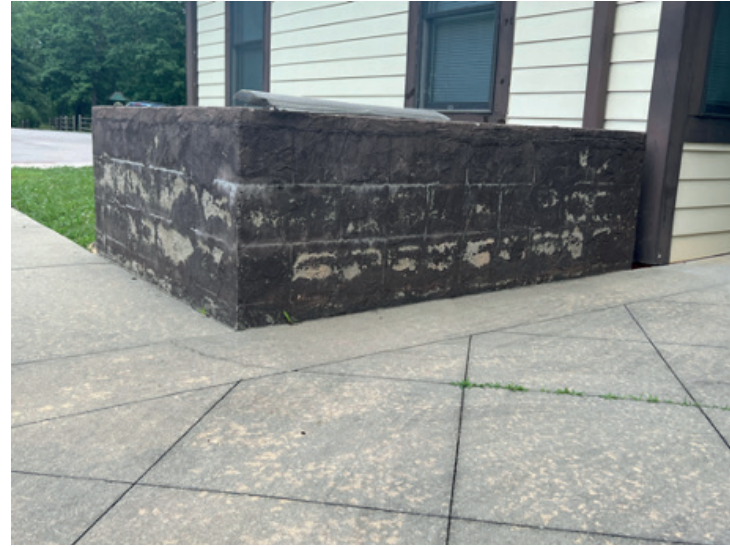
Front, brick wall, left
