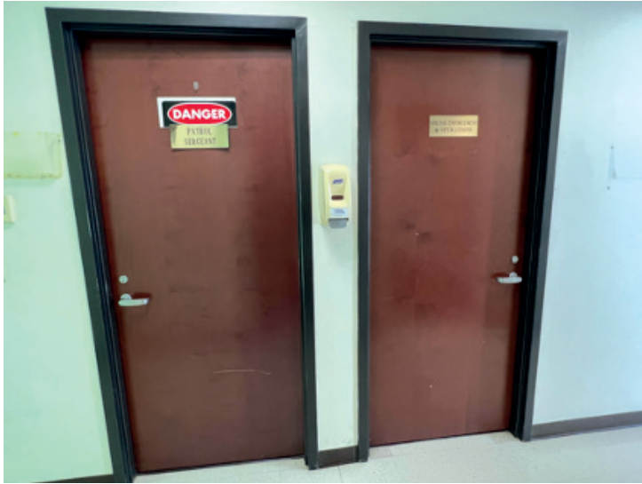
Existing Signage on Doors (111)
