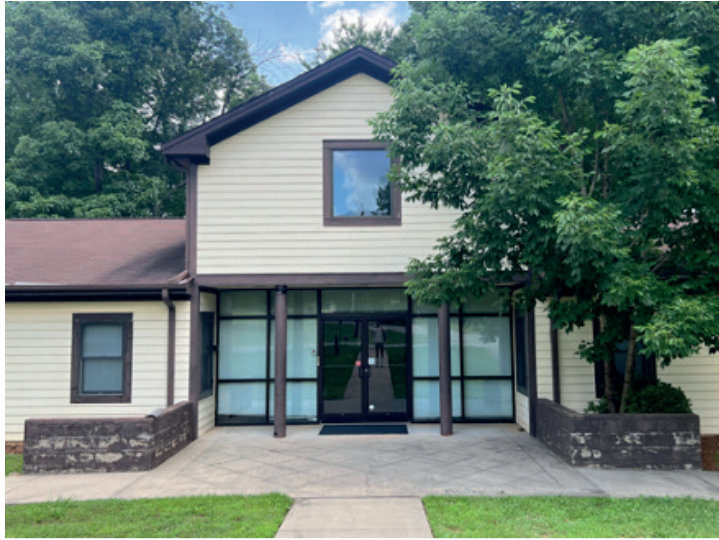
Front of building
