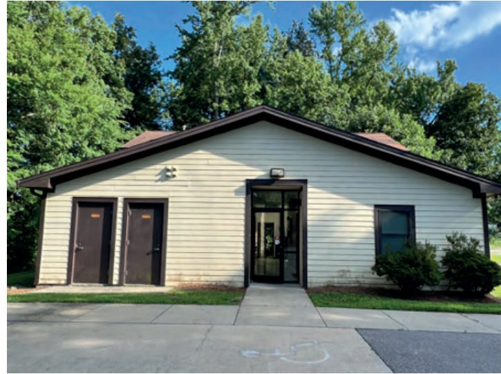
Side, view from parking lot
